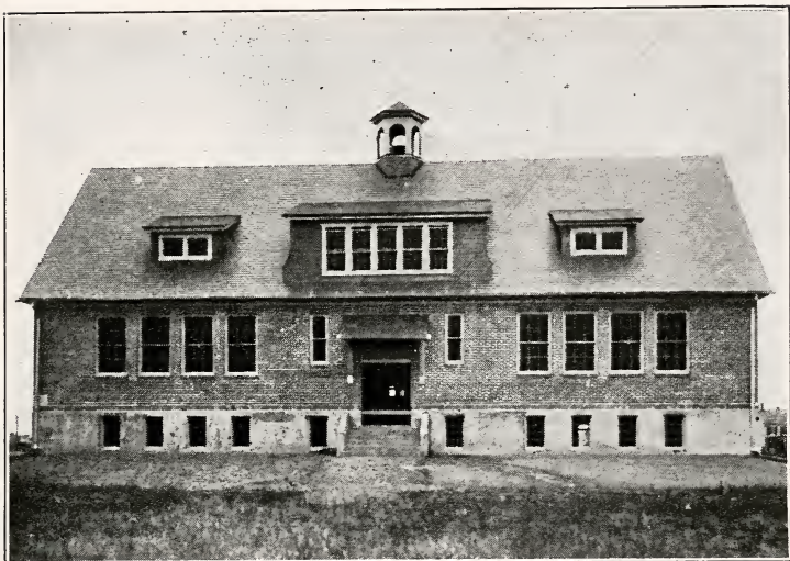
ROCK HALL HIGH SCHOOL—1915.
